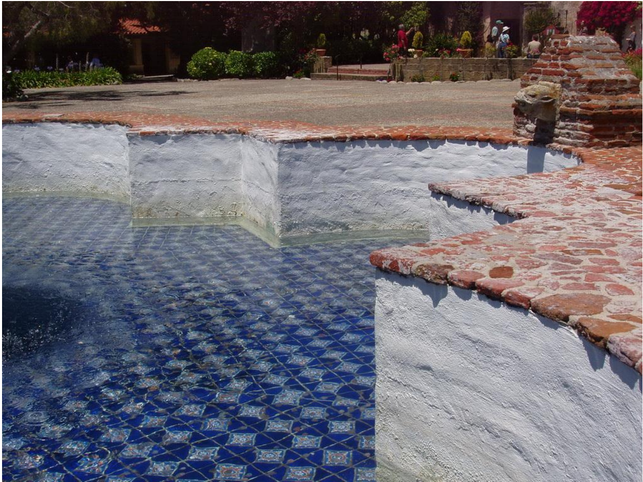
Detail of fountain basin with blue tile, stucco walls and wide brick cap. (Chris Pattillo, June 2010)
